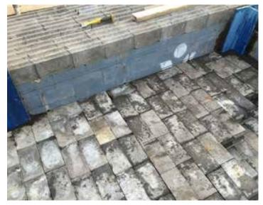
The VeriShield block is continuously laid to the thicknesses and coverage as specified in the drawings. VeriShield grout is used as necessary to fill any voids or gaps.
