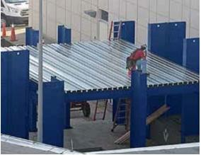
Once the outer ring of horizontal support beams is set, the additional horizontal support beams can be craned into position. Place and connect the horizontal beams to each pair of columns first.
