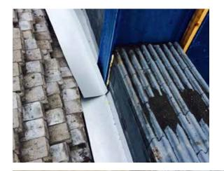
It is important to prevent any grout from slipping through any cracks down into the room below. A simple fix is to place thin strips of sheet steel over the gaps and then place the VeriShield block and grout. This will result in a clean transition between the blocks and the VPACs.
