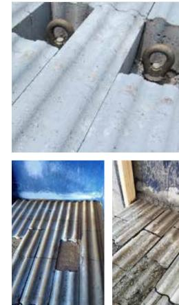
Each VPAC is transported via four lifting lugs. Once in position the lifting lugs must be removed for reuse. This will leave an opening in the VPAC approx. 5" x 5" x 5", which must be filled prior to the placement of the next layer of VPACs.
