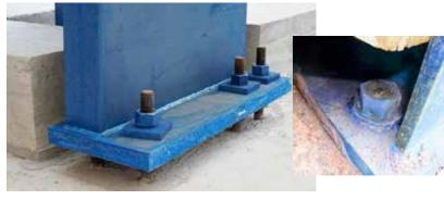
Columns are leveled and trued by turning the appropriate bolts and tightening to the specified torque. It is recommended that after leveling and tightening, the bolts be welded in place to avoid loosening.
