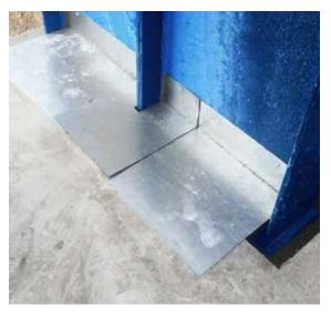
Following column placement, the bases of the columns are grouted to fully cover the attachment bolts. Column areas fully surrounded by the concrete slab can be simply filled with grout. Other areas should be formed up as necessary.
