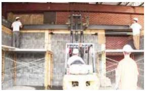
The grout is smoothed and readied for the insertion of the bearing plate anchor bolts.
