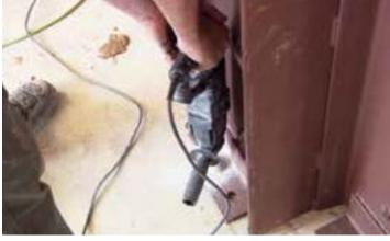
Door frame(s) shall be bolted to floor slab according to Veritas drawings. Typical embedments are 19mm (3/4") dia. HILTI H.A.S. min. 152mm (6") embed. After drilling mounting holes, fill with HILTI HY200 injection adhesive and insert bolts. Allow 24 hours. for curing before securing frame to anchors.
