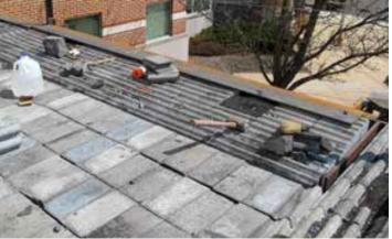
Levels of roof shielding and walls should match (unless otherwise specified in Veritas drawings), and all gaps filled with VeriShield grout.
