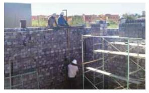
Voids are then filled with grout to fully encase the pipe within the shielding.
