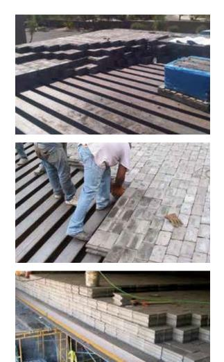
Install VeriShield block in the locations and thicknesses as indicated on the Veritas drawings.
