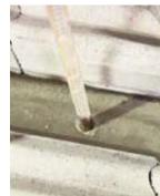
Locations for vertical rebar placement are measured out and clearly marked according to the drawings. Size and type of rebar will be specified (typically #6 rebar).
