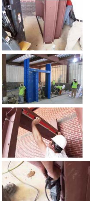
To ensure the door frame is level and plumb it is strongly suggested that the door width be measured at a least three points - the bottom, the middle and the top as shown in the diagram below. The frame should be square and plumb.
