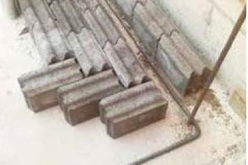
Once the vertical rebar is set, additional rebar is added horizontally to reinforce the horizontal bond beams. Where sections of rebar overlap, a minimum of two feet of overlap is required and overlapping sections of rebar must be tightly wired together every 12 inches in distance. All corners and intersections shall have a minimum two-foot rebar overlap.
