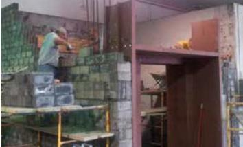
VeriShield block is laid up to the door frame and grout added to fill any voids. Subsequent layers are laid leaving space around the embedment studs welded to the frame. These spaces are filled with grout, firmly embedding the studs within the wall shielding
