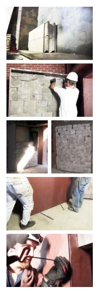
While the door remains on the pipes, or other support at the middle and ends of the frame, begin loading block starting on the strike side of the door starting with a full block. Keep block tight to door shell. Stagger pattern every two courses, keeping block tight together. Cut blocks as necessary to fill door shell as completely as possible.
