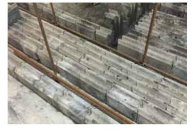
Vertical rebar is inserted into the holes and set as deeply as possible. Allow epoxy to cure prior to attaching horizontal rebar. Sections of rebar shall be oriented in the middle of the horizontal bond beam.
